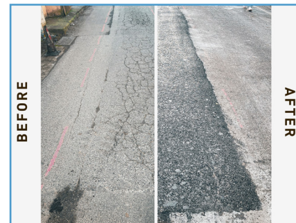
Above: The machine recovers and reuses 100 per cent of the on-site material.
