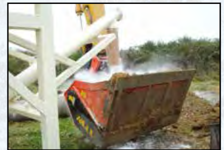
Stabilising soil with lime
