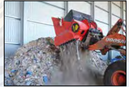
Crushing demolition waste
