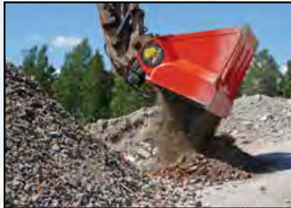
Crushing bricks / black top asphalt
