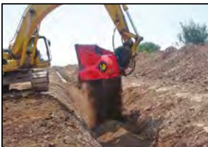
Pipeline padding/back filling
