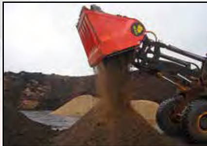
Mixing top soil and sand
