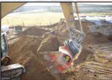
Stabilising foundation layers
