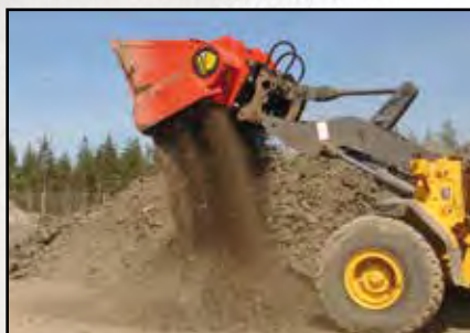
Aerating contaminated soil compost
